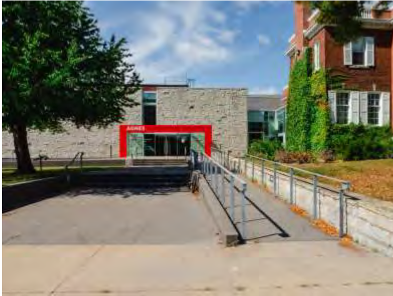
Image: View of Agnes's Main Entrance off University Avenue and location of accessibility ramp.
